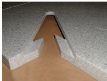
(9) Remove template, counter is now ready
